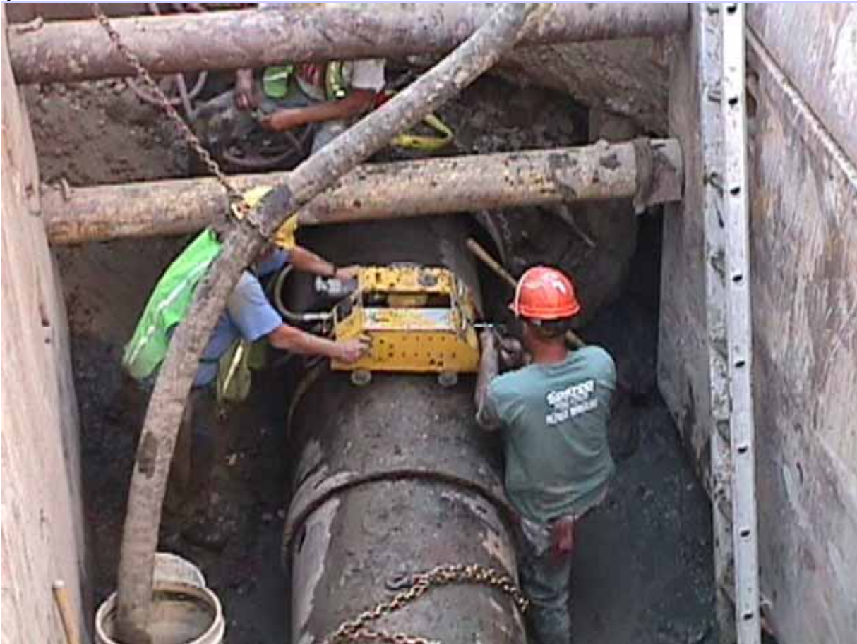
Work on water distribution main
