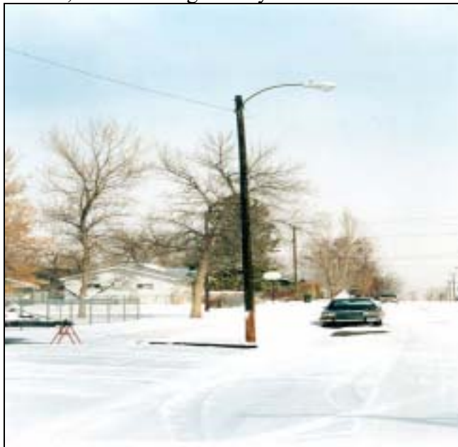
70 Watt Single Wood Pole O/H
